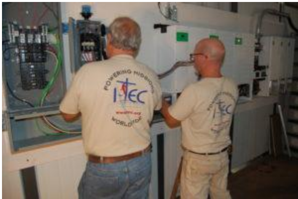
Power Pac under construction
